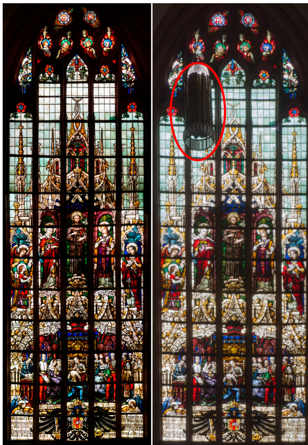
Figure 10. Comparison of the image of the stained glass composed from the images captured by an onboard camera of an unmanned aerial vehicle (left) and static camera mounted on the tripod at the floor of the temple (right). Besides a worse quality of the image with respect to capturing real-world dimensions of an object, the image captured by a static camera includes an area occluded by the chandelier (highlighted by a red ellipse), which is inevitable when capturing images from the ground.
