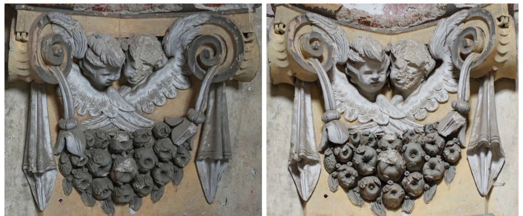
Figure 6. Comparison of the image taken by the onboard camera (left) and the image taken by the handheld camera from the ground (right). Although an object is located only 12 m above the ground, the difference in captured surfaces between the image captured from the same height and the image captured from below is significant.
